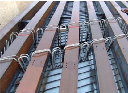
Figure 26: Installation of reinforcement on site [U11]
