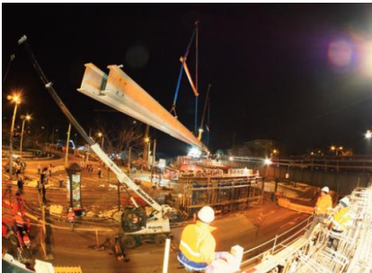
Figure 25: Installation of the rolled iron girders [U11]
