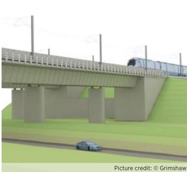
Figure 15: poor abutment design
